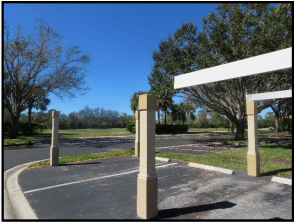
Carport with missing roof
