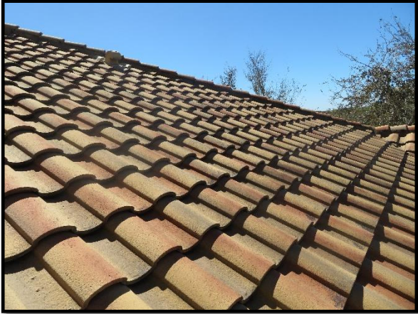
Closeup of concrete tile roof
