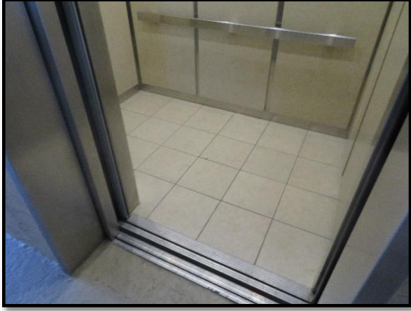
Elevator cab finishes
