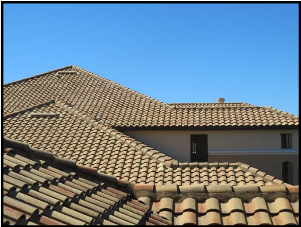
Concrete tile roof
