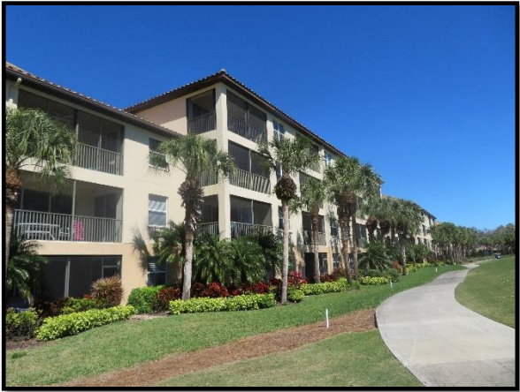
Rear elevation overview
