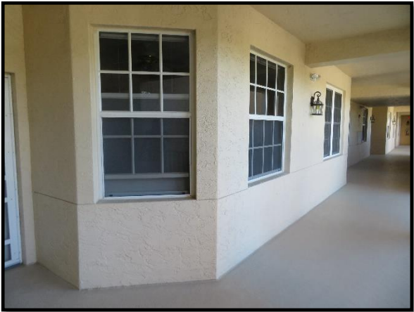
Breezeway paint finishes
