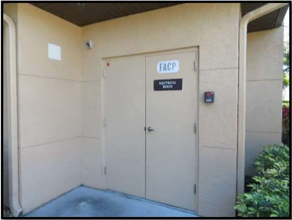
Common mechanical room door
