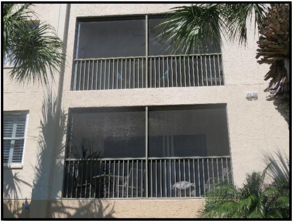
Rear elevation balconies
