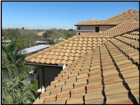
Closeup of concrete tile roof
