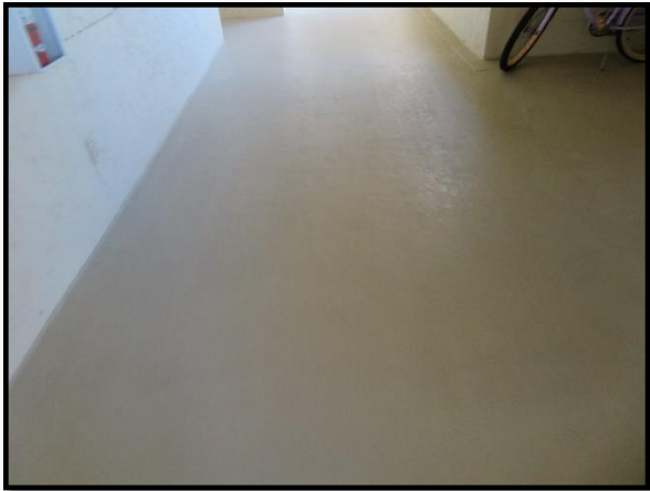
Breezeway with floor coating
