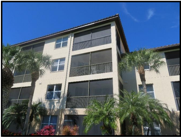
Rear elevation balconies
