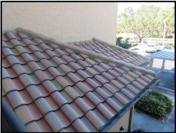
Closeup of concrete tile roof
