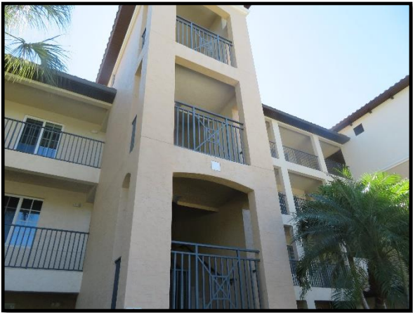
Exterior paint finishes
