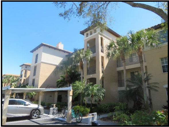
Front elevation overview
