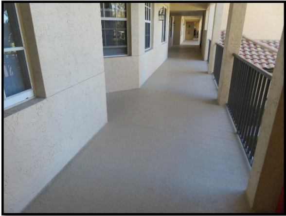
Breezeway with floor coating
