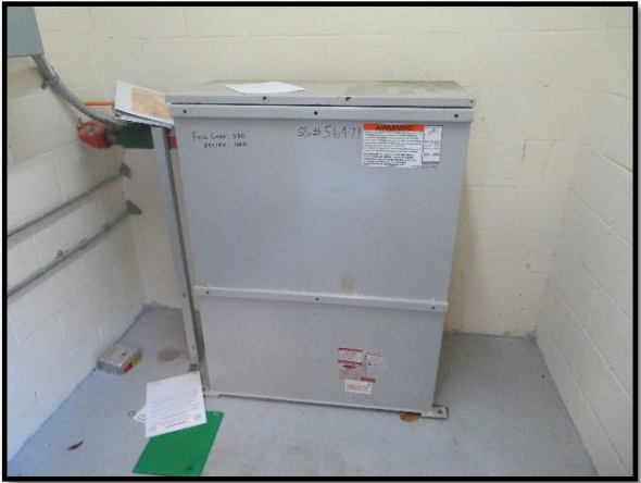
Elevator hydraulic pump
