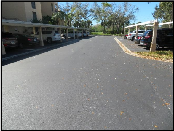
Asphalt pavement overview
