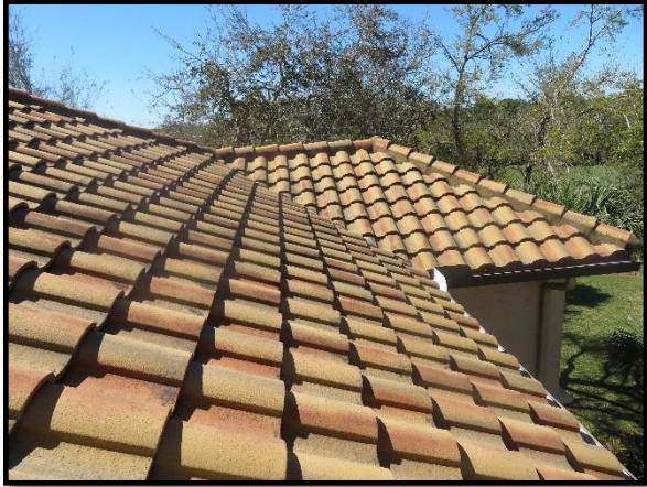
Closeup of concrete tile roof
