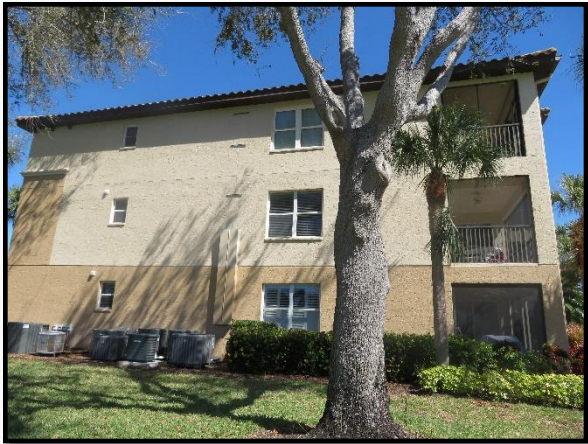
Side elevation overview
