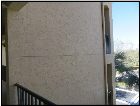
Exterior paint finishes
