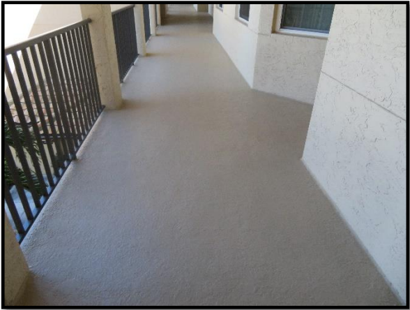
Breezeway with floor coating
