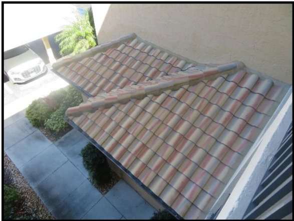
Closeup of concrete tile roof
